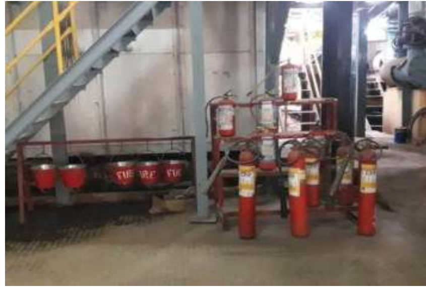
Photographs of firefighting arrangements
